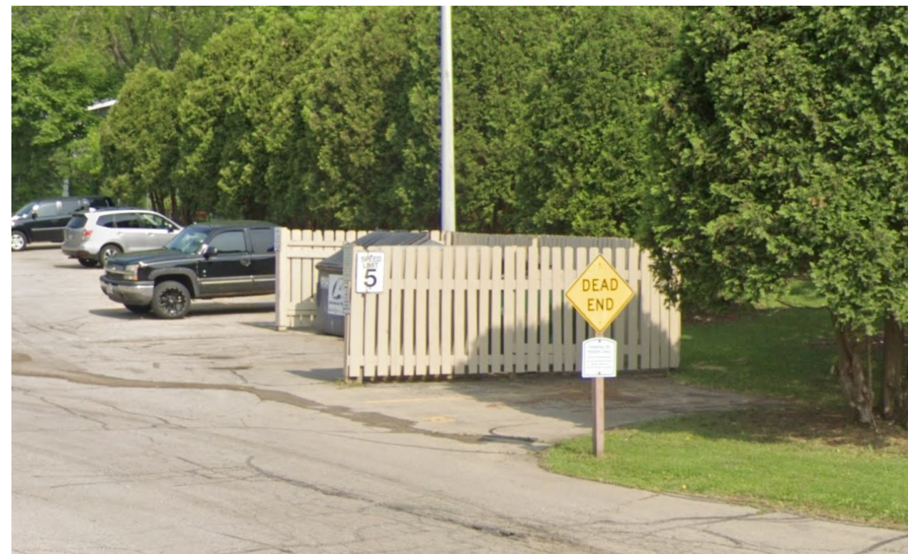
5A/A100 EXISTING TRASH ENCLOSURE
