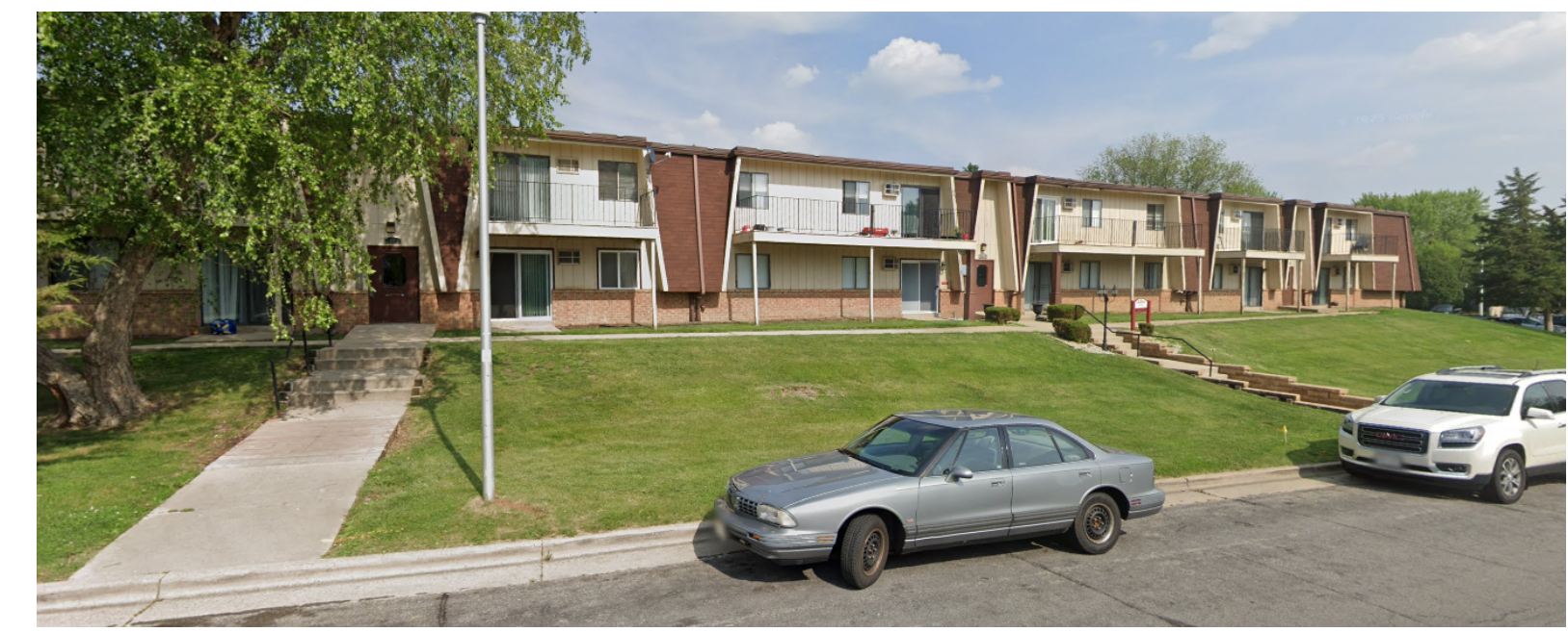
2A/A000 EXISTING - ALONG RED ARROW TRAIL 2
