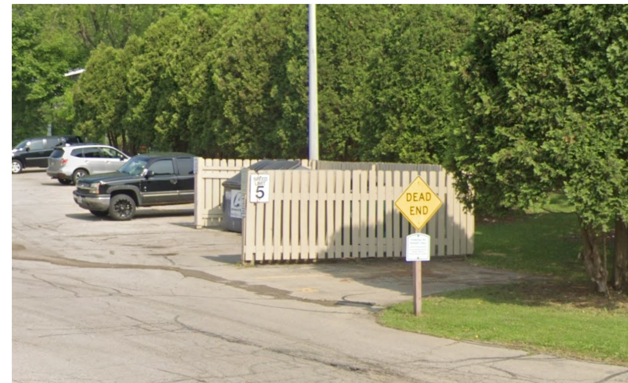
5A/A100 EXISTING TRASH ENCLOSURE
