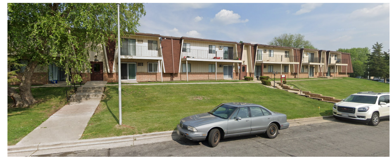
2A/A000 EXISTING - ALONG RED ARROW TRAIL 2
