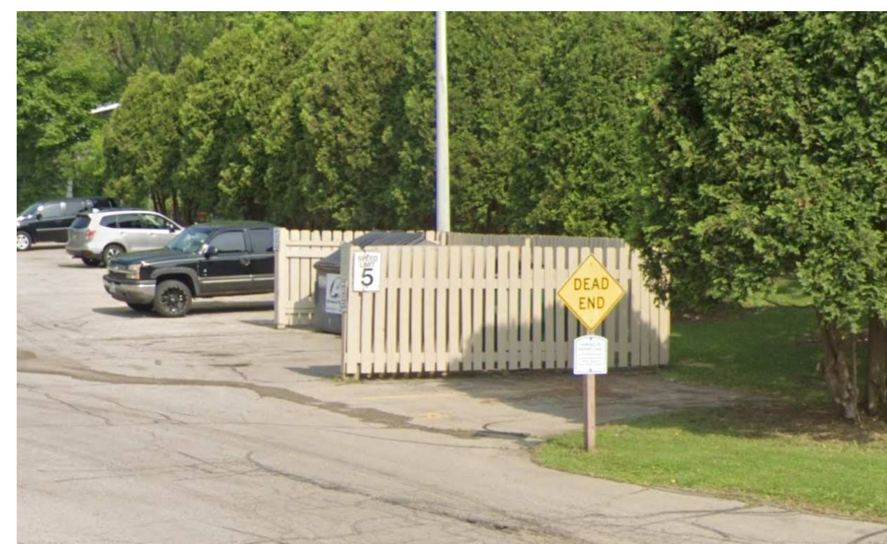
5A/A100 EXISTING TRASH ENCLOSURE
