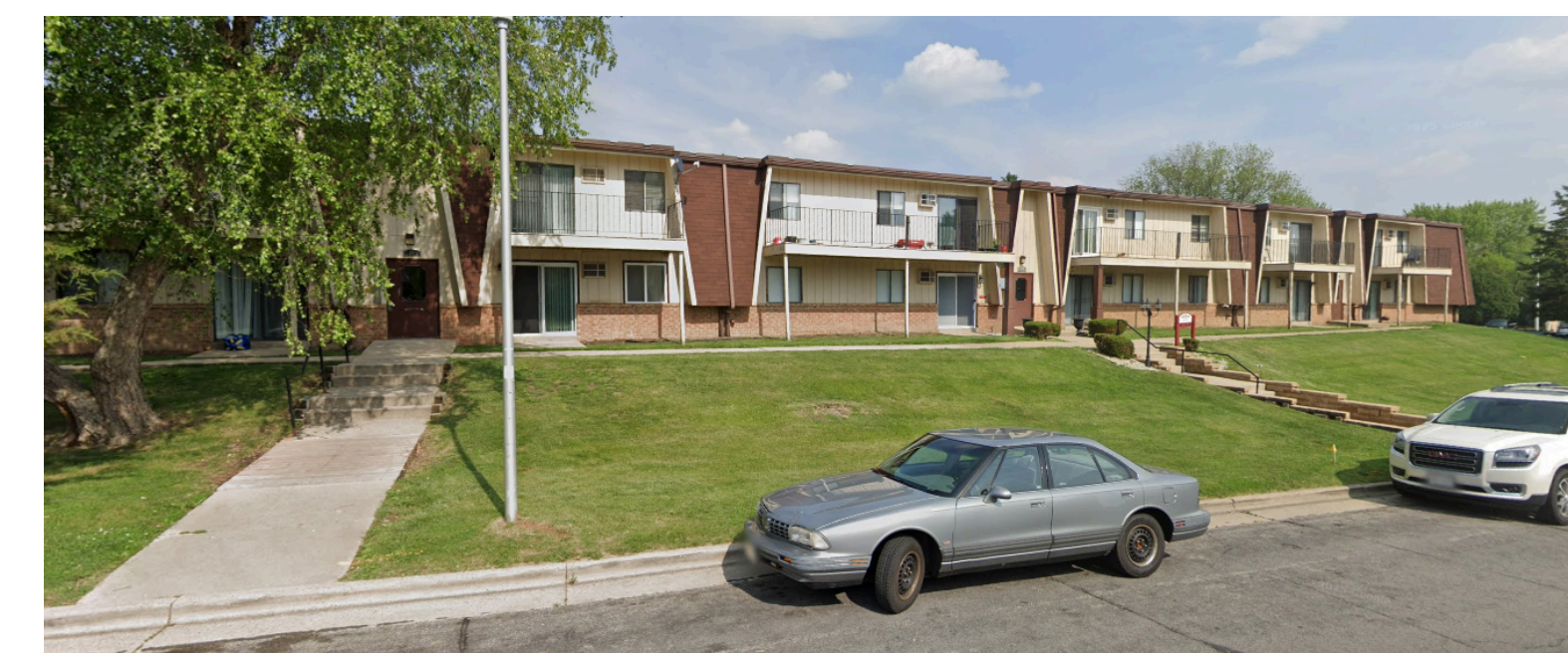
2A/A000 EXISTING - ALONG RED ARROW TRAIL 2
