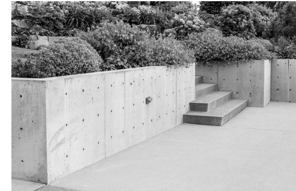
CONCRETE WALL - ARCHITECTURE FINISH
