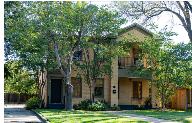
Small multi-unit housing can fit seamlessly into the neighborhood.
